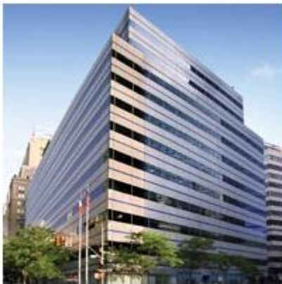
Three city agencies are located on floors 6 through 9 at 75 Park Place.
